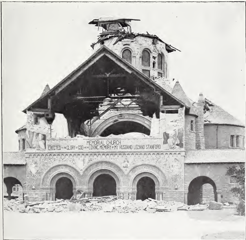
J. COLLAPSED TOWER AND GENERAL EARTHQUAKE WRECKAGE, MEMORIAL CHURCH, LELAND STANFORD JUNIOR UNIVERSITY.
